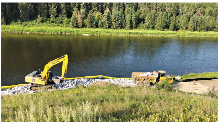
Slope repair involved reinforcing the river bank with class 1 and 2 'rip rap' rocks.
